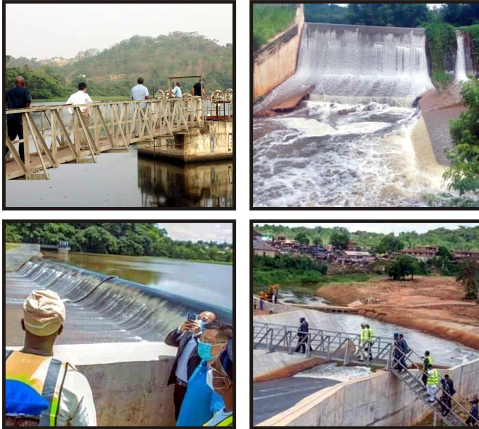
Oke-Badan at Eleyele Reservoir
